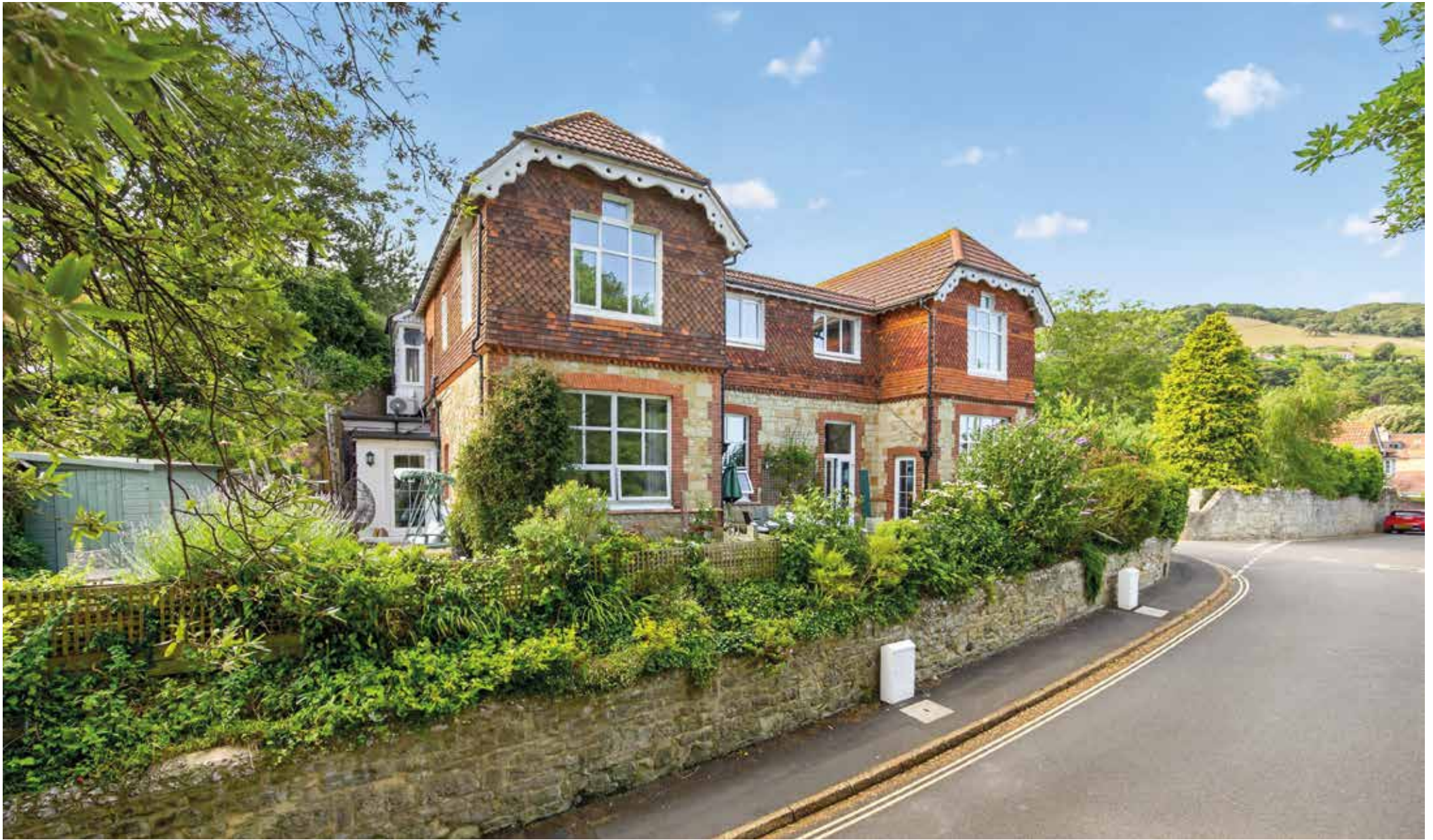
Cornerways 39 Madeira Road | Ventnor | Isle of Wight | PO38 1QS
